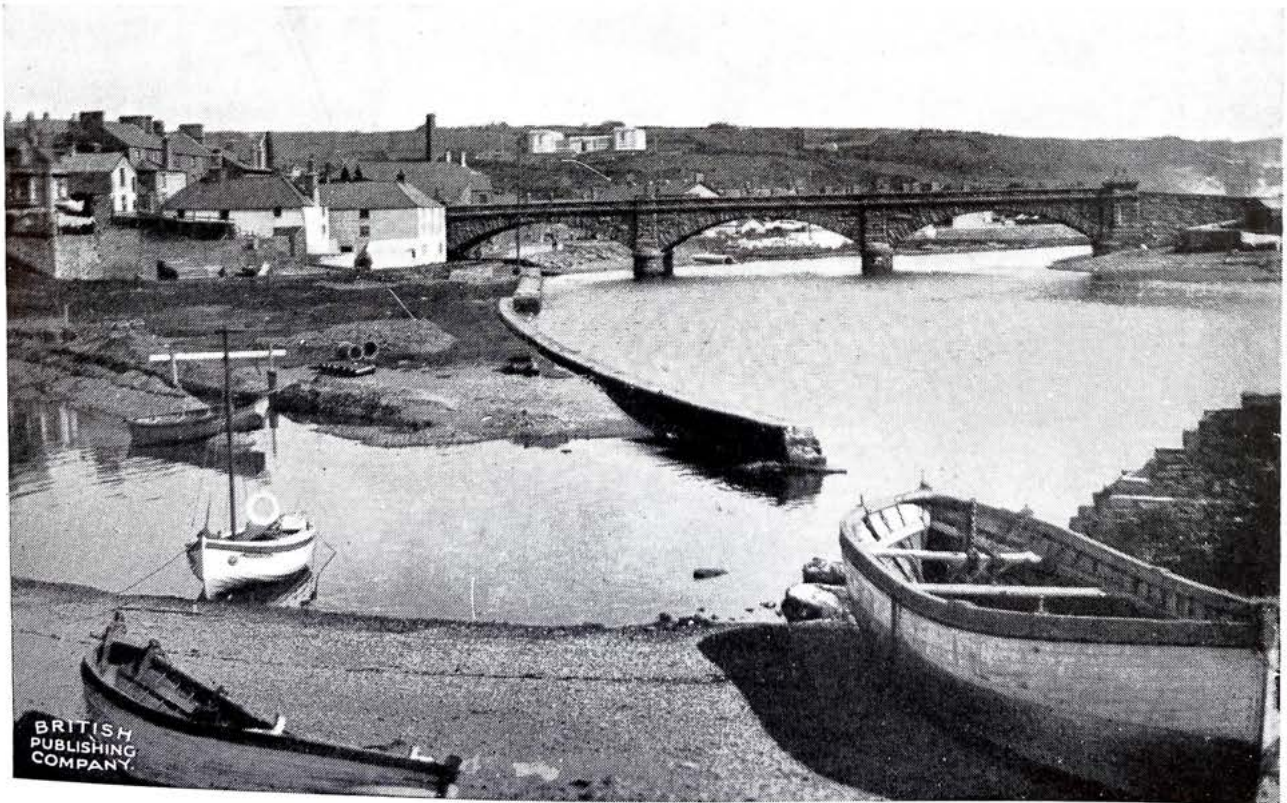
TREFECHAN BRIDGE FROM HARBOUR AND NATIONAL LIBRARY ON THE HILL.
